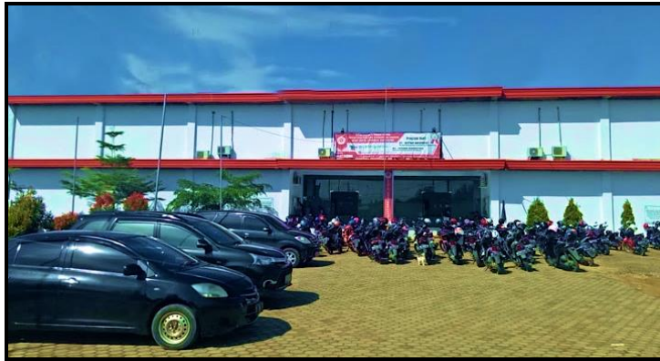
Gambar 3. Gedung Kampus ITBADCC PSDKU Kotabumi
